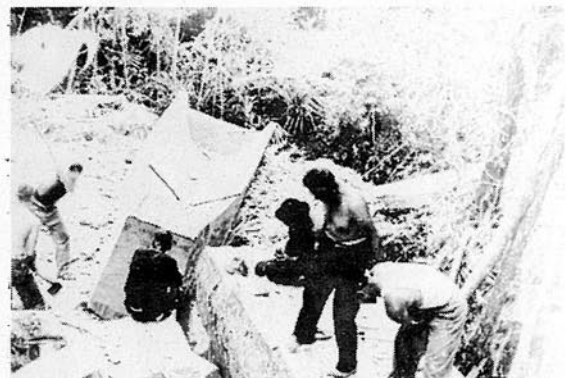
Further work before transporting.
