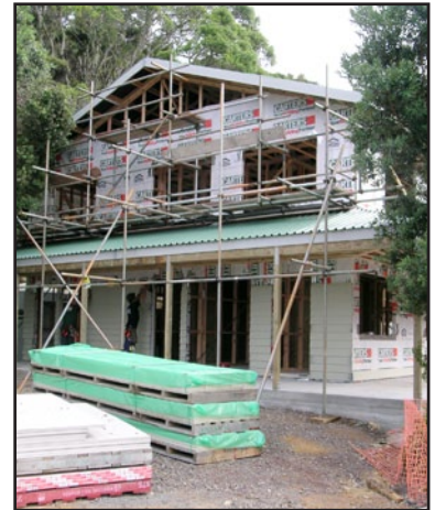
New Marina building, under construction.
